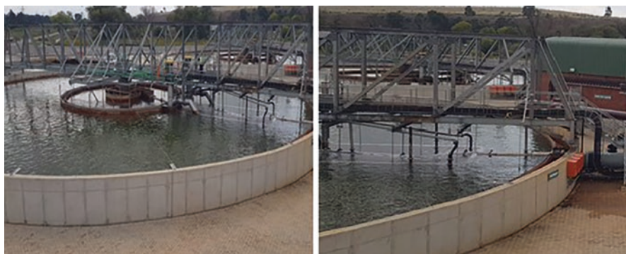
Fig. 4.11 Settling tanks. (Photographs by researcher)
