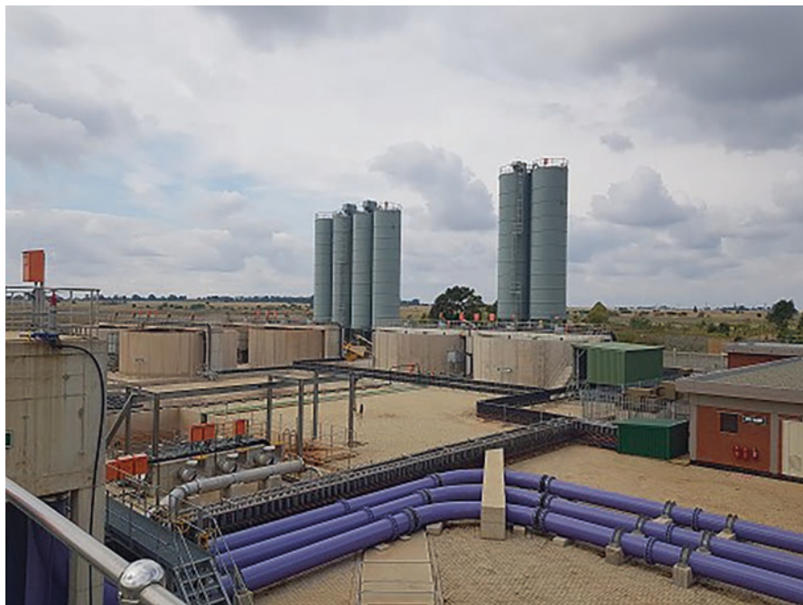
Fig. 4.7 Silos filled with lime. (Photograph by researcher)
